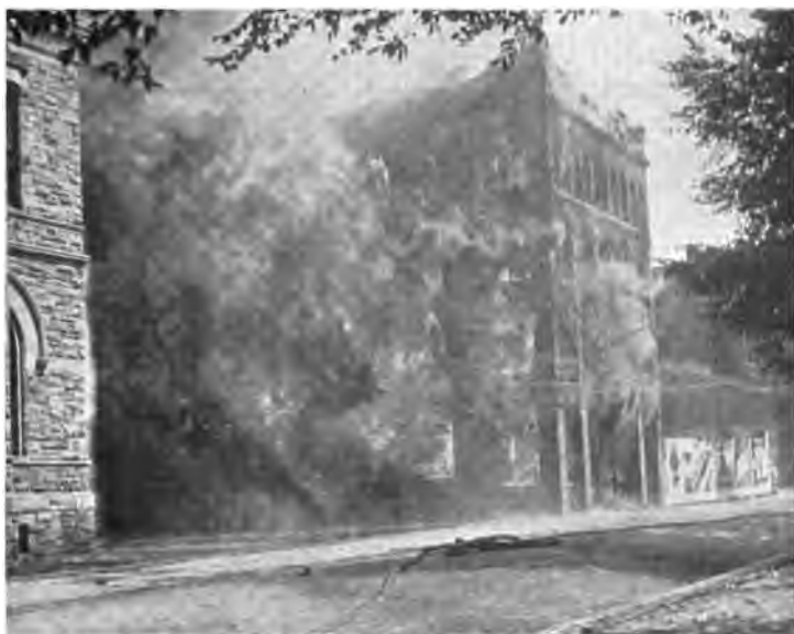
Fig. 1. Binghamton Clothing Company Building, Ten Minutes after Fatal Fire started.*
